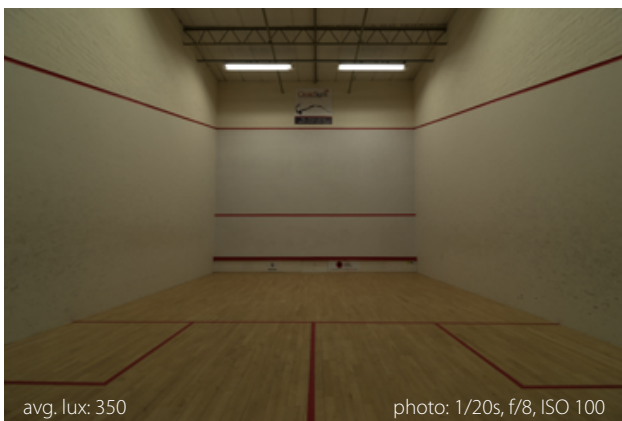
Before: Court no. 1 illuminated with 12 x 77W Fluorescent Tube Lights
