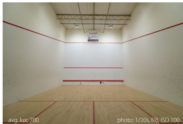
After: Court no. 1 illuminated with 6 x 130 Eco-Range Squash 130 fixtures
